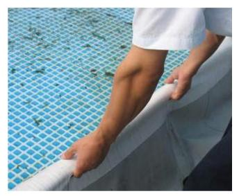
**Step 3:** Grasp the end of the tube and rotate it from side to side while pulling the beam out of the sleeve
