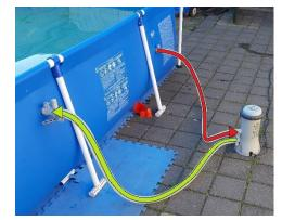
**Tip:** Do not connect extra hoses to your pump. This will increase the path to and from the pool and requires more water pressure. This will reduce the performance of the pump.
